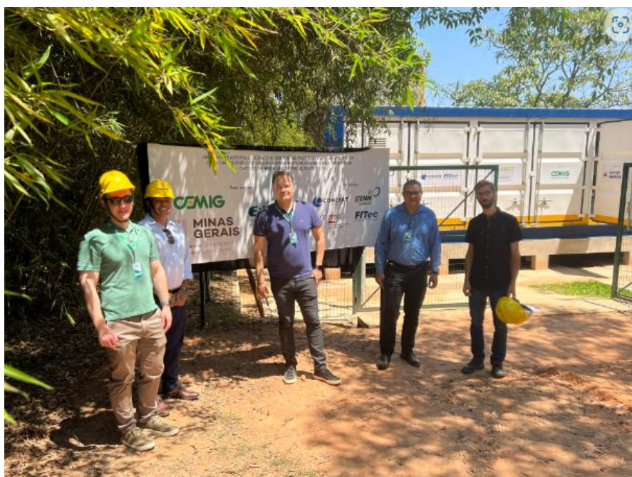
Image of representatives from Cemig's team getting to know the storage pilot plant
